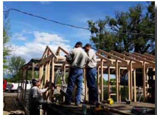
Chicken Coop Construction
