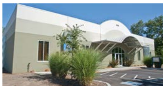
New Chico Substation
